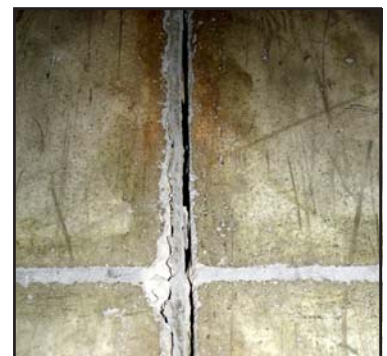
Deteriorated wheels, excessive surface wear and spalled joints are telltale signs of an owner who is not "floor conscious."
