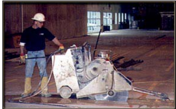
Traditional “wet cut” saws require sufficient slab cure to support the saw's weight.
