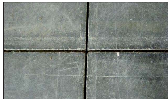
Minor edge chipping is not unusual on new floors to be filled. Chips wider than 1/16th" (2mm) should be “squared off” prior to filling.
