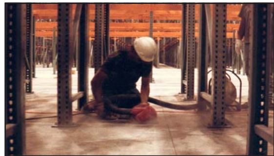
Joint preparation (cleaning) is critical in ensuring long term filler durability. The use of dry-cut type, vacuum equipped saws to clean joints is the preferred method of preparation.
