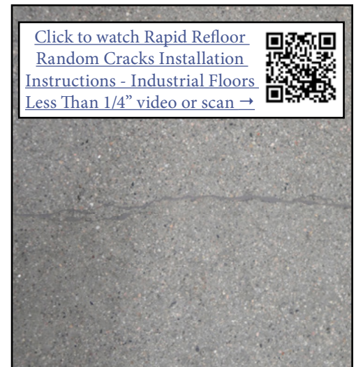
Step 3 Vacuum crack thoroughly. Crack must be dry prior to application of product.
