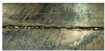
Joint deterioration is gradual but inevitable when an inferior filler is chosen or if a filler is installed poorly. As the deterioration increases, the cost of repairs increase and your productivity decreases.
