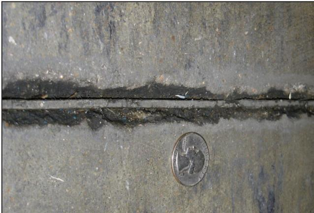
*Correction:* Remove existing filler completely, clean joints properly as outlined in Metzger/McGuire Installation Guidelines and refill properly.
