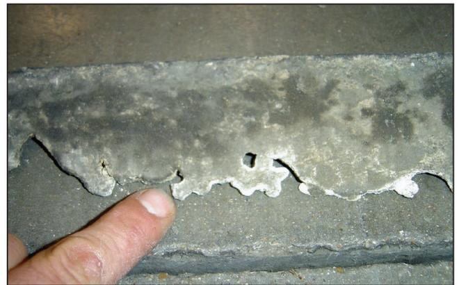
*Correction:* Remove existing filler completely, clean joints properly as outlined in Metzger/McGuire Installation Guidelines and refill properly.
