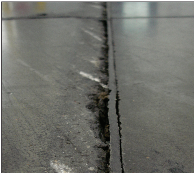
Curled slab panels create impact points for material handling vehicle wheels, and joint edges along curled panels can quickly deteriorate if left uncorrected.
