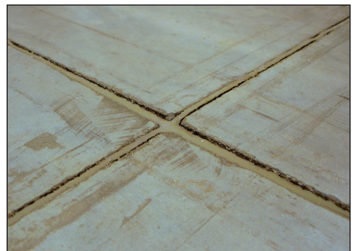
Curled or rocking slab panels can compromise the ability of the filler to provide proper edge protection.
