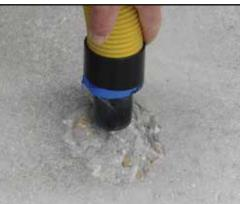
Step 2 Clean out any remaining debris or loose elements. Vacuum thoroughly. Repair surface must be dry.
