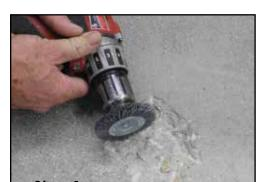
Step 1 Remove any unsound or loose concrete. Run drill with Nyalox or soft wire wheel over defects twice (in opposite directions). If bolt is present pound/cut down to allow 1/2" material cover.
