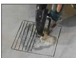
Step 1 Make cuts with blade or chip out section at outer edges of spalling, 1/2" deep (minimum) to 3/4" deep (preferred). Creating a vertical edge.
