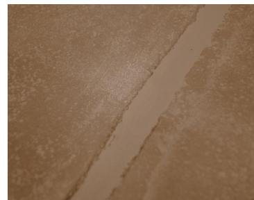
Finished repair after razoring
