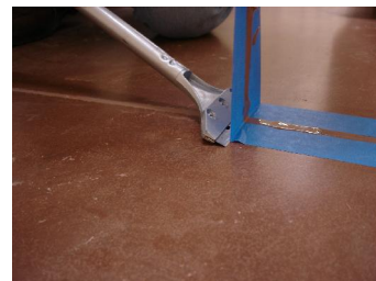
After RS-88's initial cure (approx. 15 mins) excess material is razored off.
