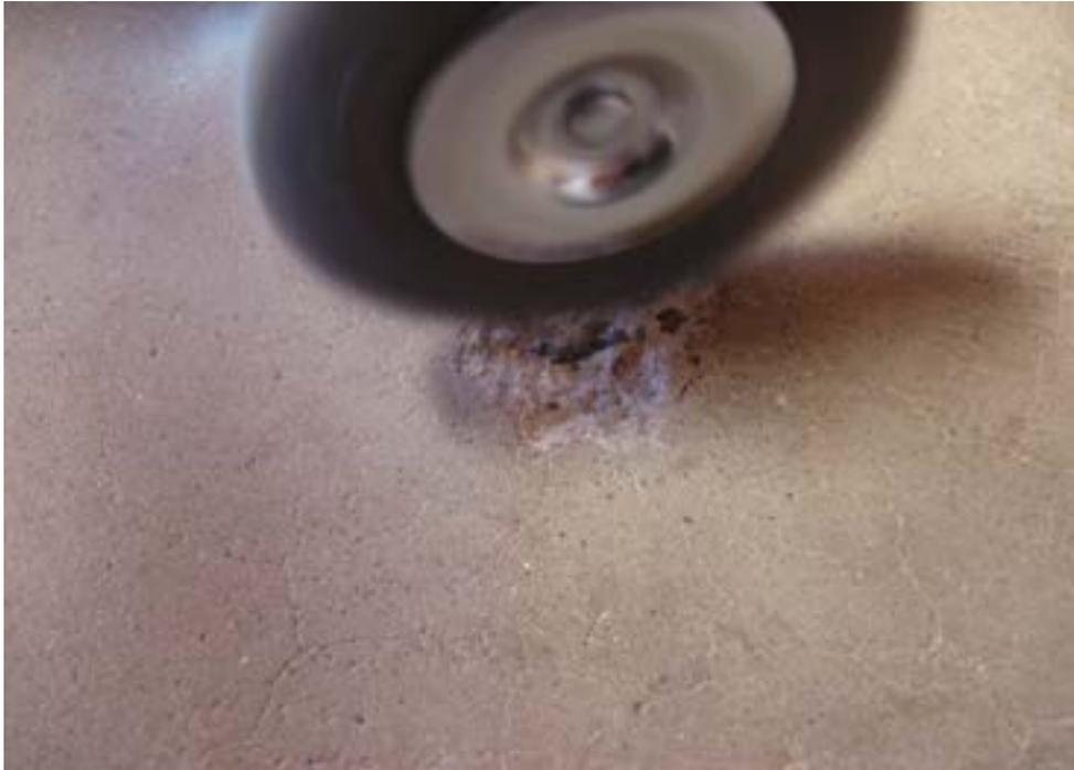
*Step 1: Clean defect of all dirt and debris using soft wire or Nyalox wheel.*
