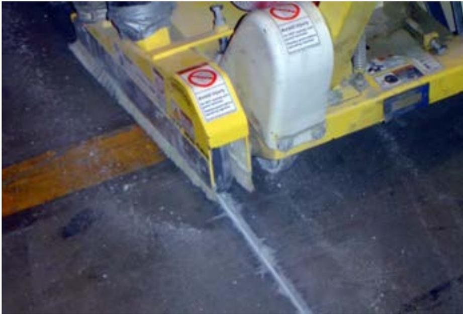
*Step 1: Saw cut behind outside of any joint edge spalling to a minimum depth of 3/4".*
