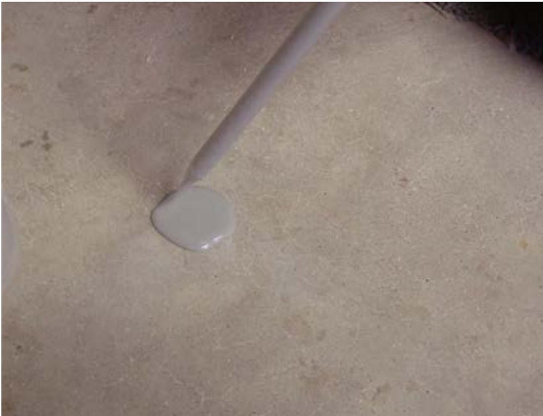
*Step 2: Slightly overfill defect with Rapid Refloor, allow to cure 30 mins or more.*
