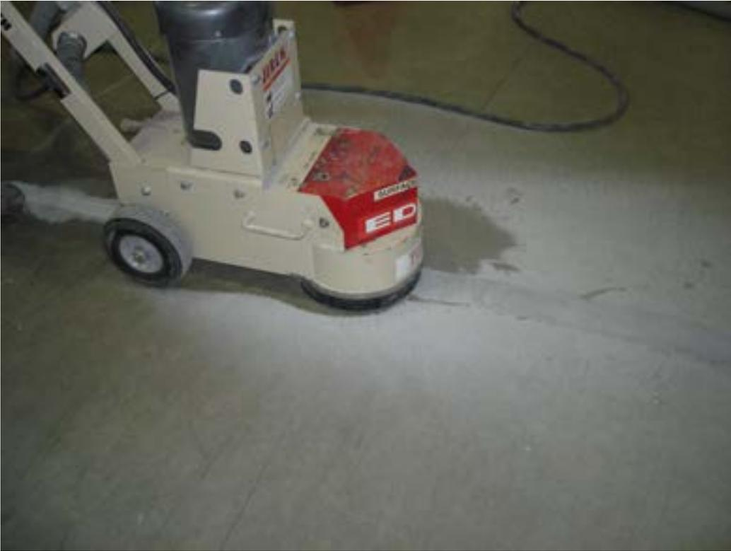
*Step 4. Allow mortar to cure into solid (2 hrs plus) and grind flush with floor surface.*
