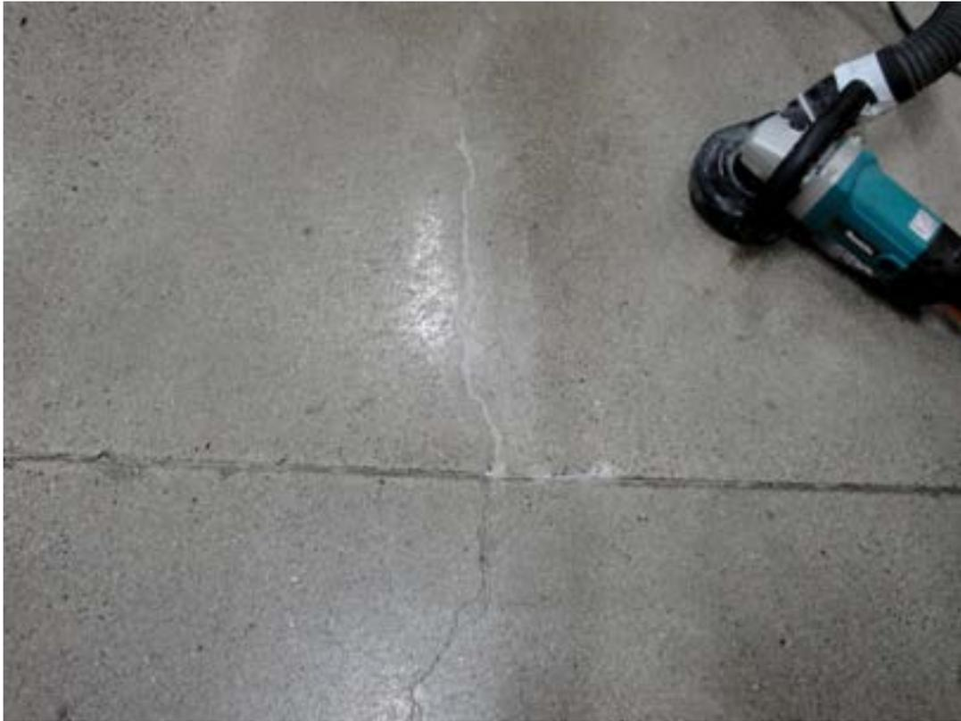
*Step 4: After material cure (approximately 30 mins. or more) grind overfill flush with floor surface using specified finishing pads.*
