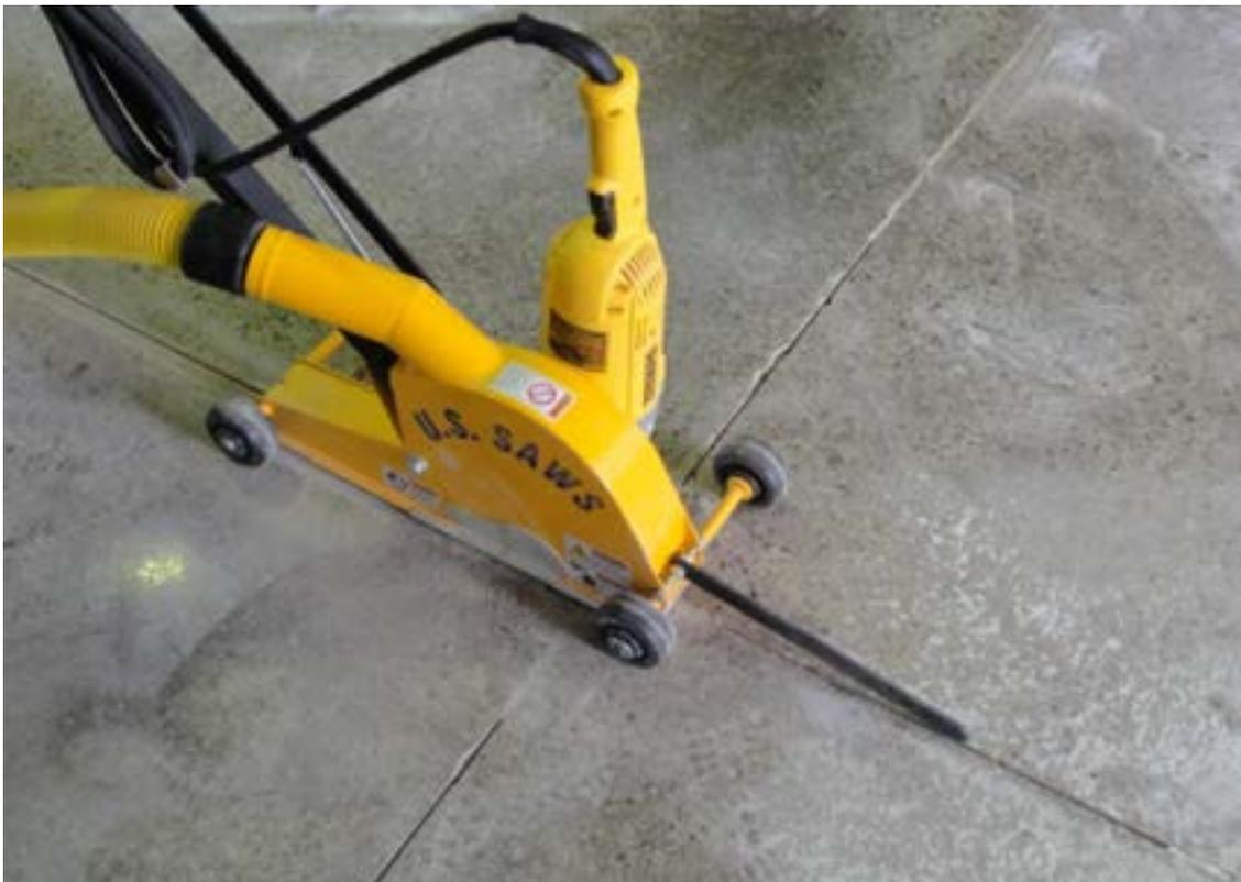
*Step 3: Re-saw cut through repair along edge of joint spall repair.*
