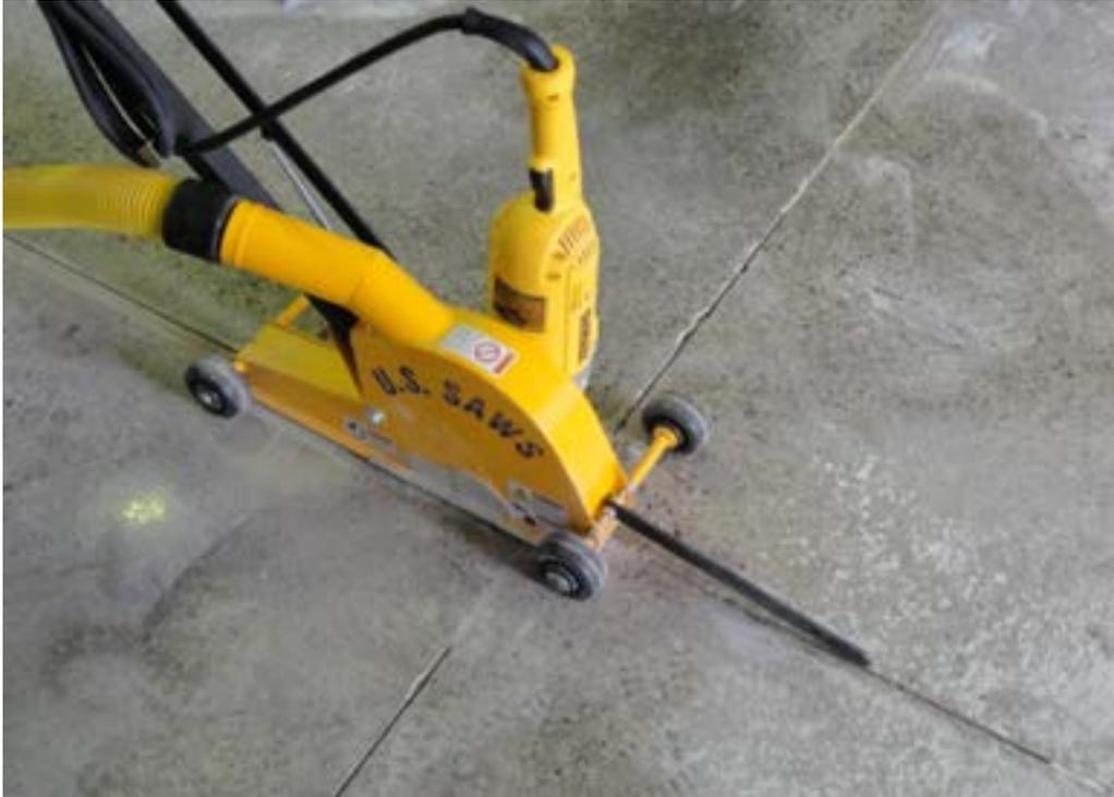
*Step 1: Saw out all existing filler to full depth of original joint.
