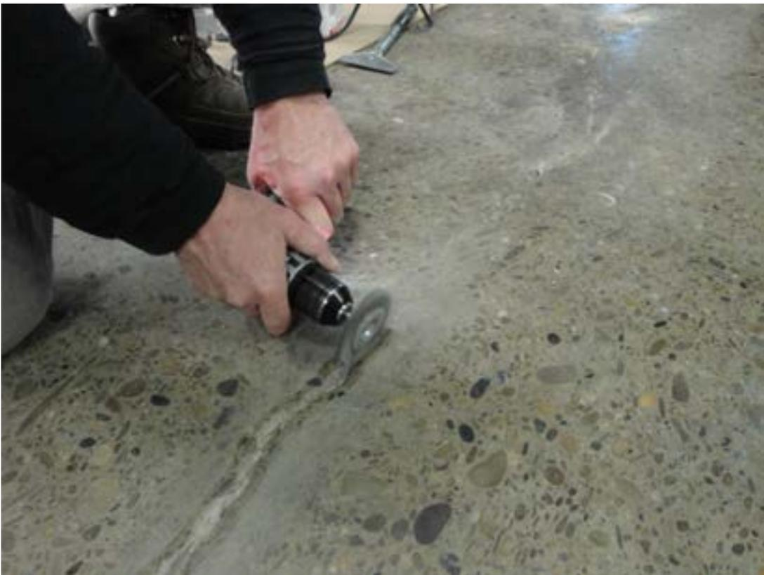
*Step 1: Chase crack using small grinder equipped with Nylalox or soft wire wheel brush.*
