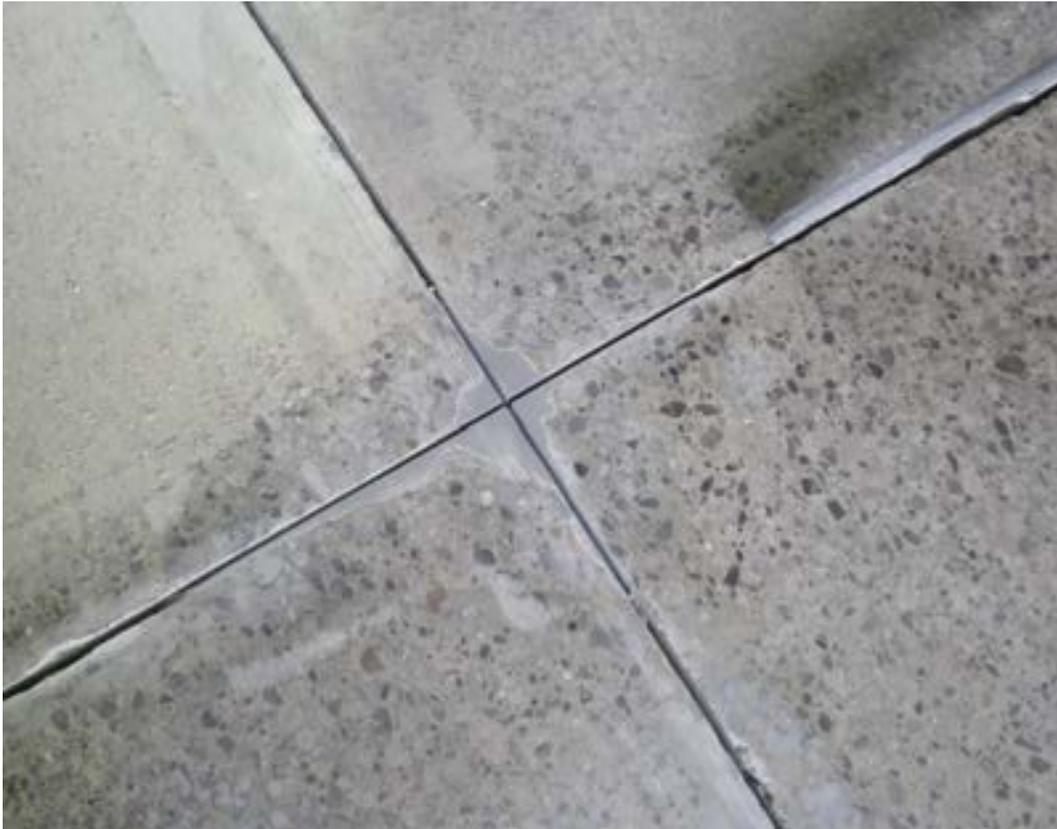
*Finished example of joint edge spall repair.*
