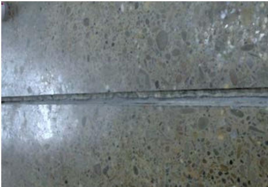
*Example of properly cleaned joint. Edges should be clean and crisp.*
