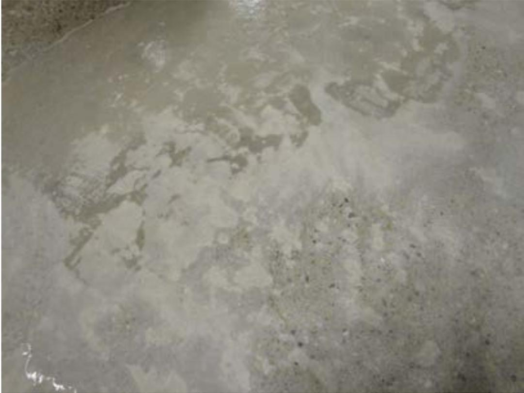
Condition After Initial Metal Grind
