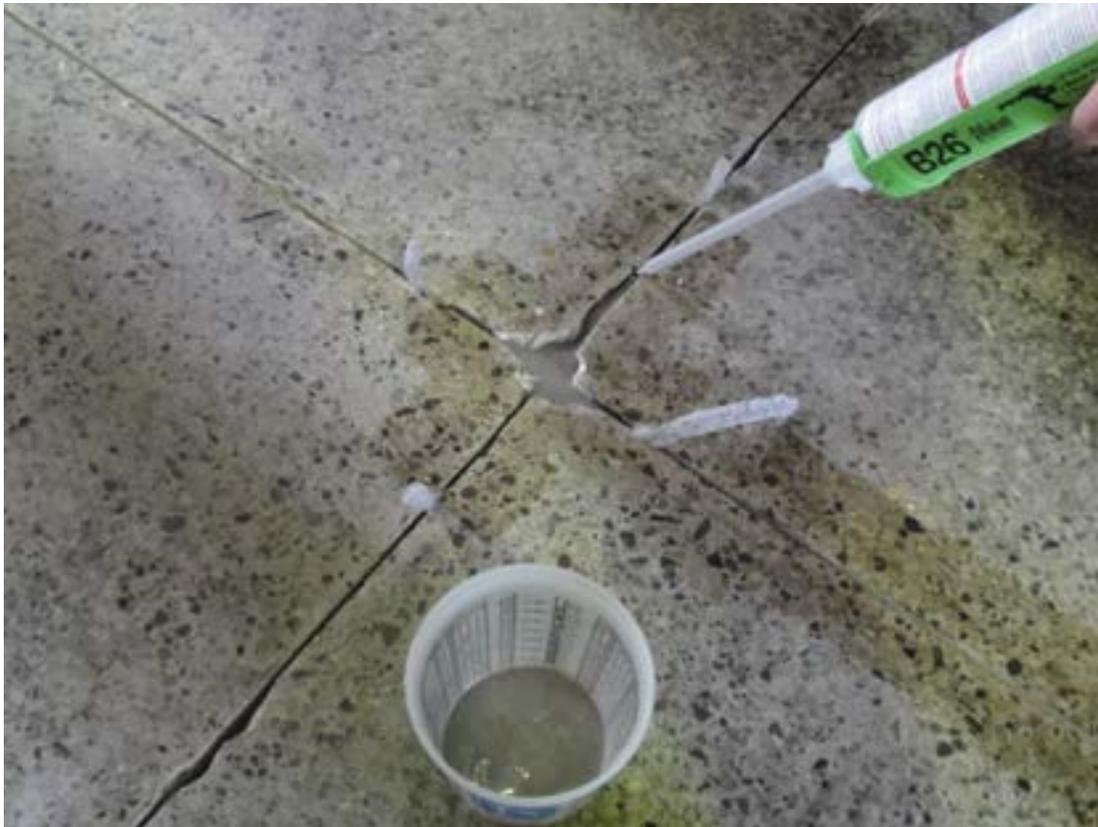
*Edge spall repair Step 1: Dam off area around edge spall. Slightly overfill with Rapid Refloor*
