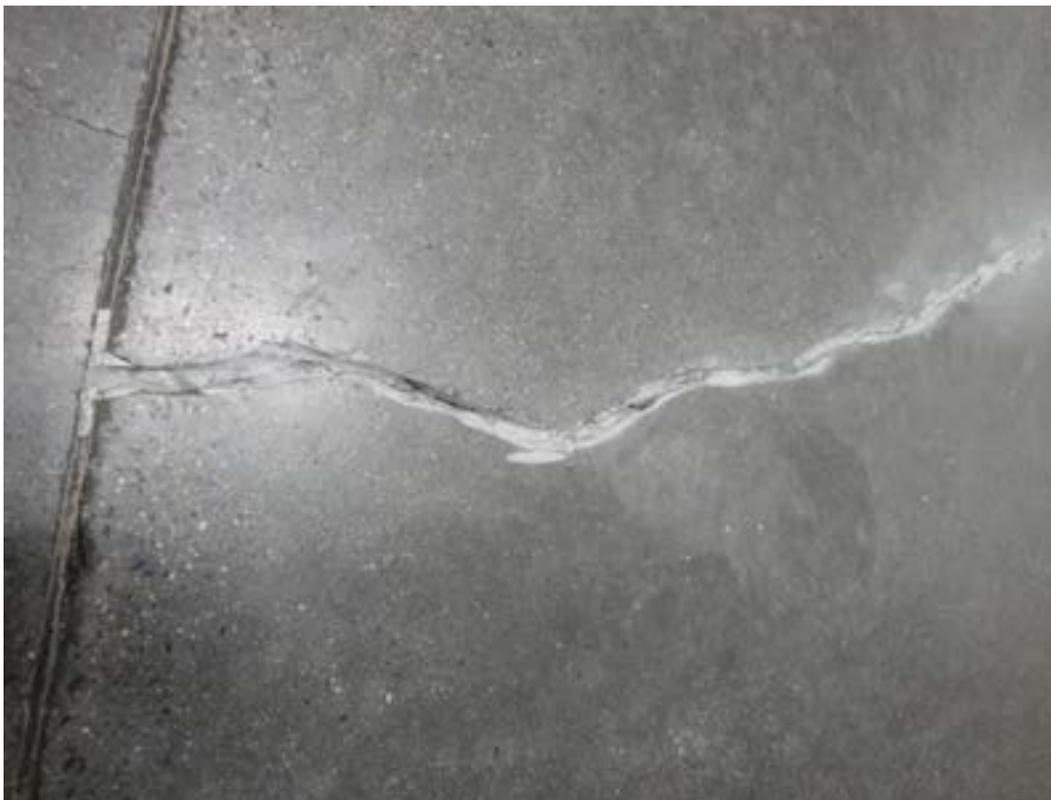
*Example of properly prepared crack. Edges should be neat and crisp; nominal depth of repair 1/2" deep.*
