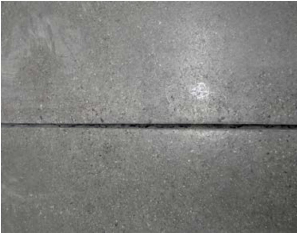
*Example of properly cleaned/prepared joint.
