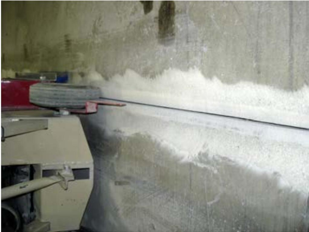
*Step 6: Saw cut along chalk line over existing joint. Cut should go completely into original joint.*
