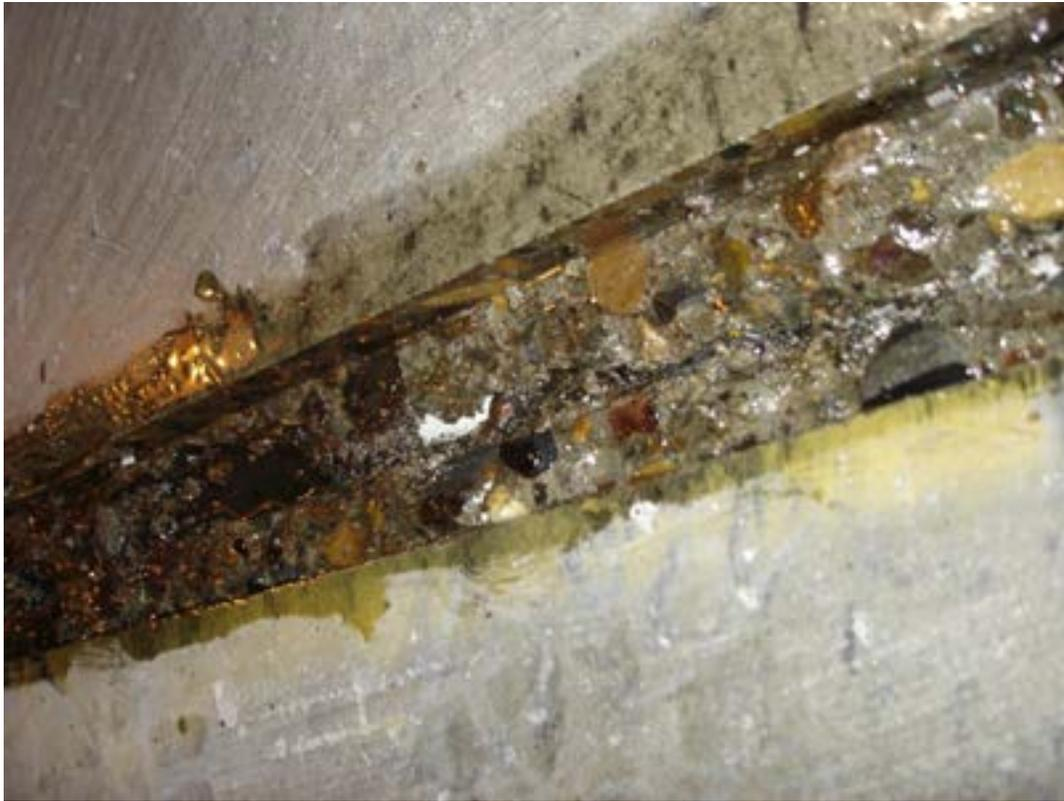
*Step 2: Prime newly cut repair channel with neat liquid Armor Hard Extreme*
