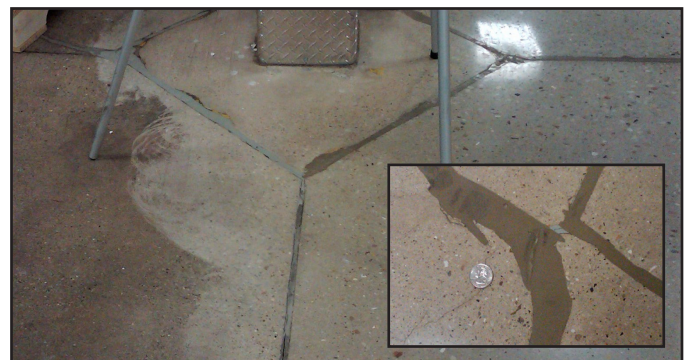
Example of poor color match resulting from matching to the existing surface prior to initial grind.
