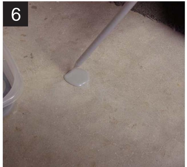
Dispense material into defect, slightly overfilling edges. **IMPORTANT:** Keep gun pointed down at all times during dispensing/moving to ensure material does not flow back into cartridge unit, which can lead to soft spots.
