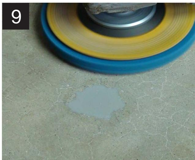
Finished profile of Rapid Refloor should be completely flush with floor surface.
