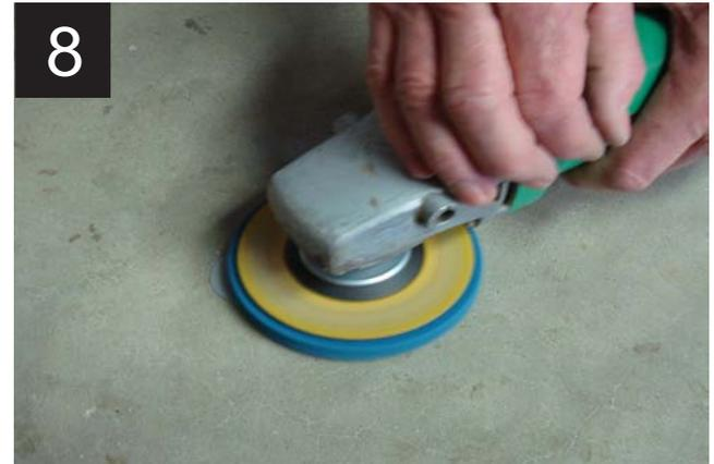
When grinding keep pad flat to the floor surface and grind off overfill until repair is flush with floor surface. Grinding at an angle will leave profile low. If material is tacky or gummy, stop grinding immediately.
