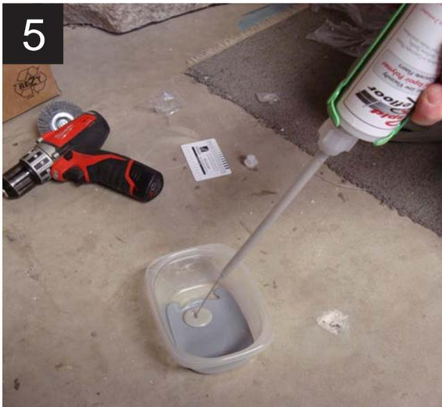
Tip gun down and dispense 2-3 waste shots into disposable container until color mix is consistent.
