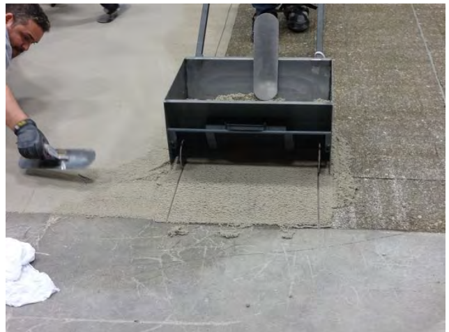
Troweling AH HDR behind the screed box
