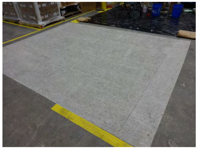
Profiled area. Edges squared up – no feather edging.
