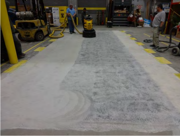
Grinding AH HDR next morning
