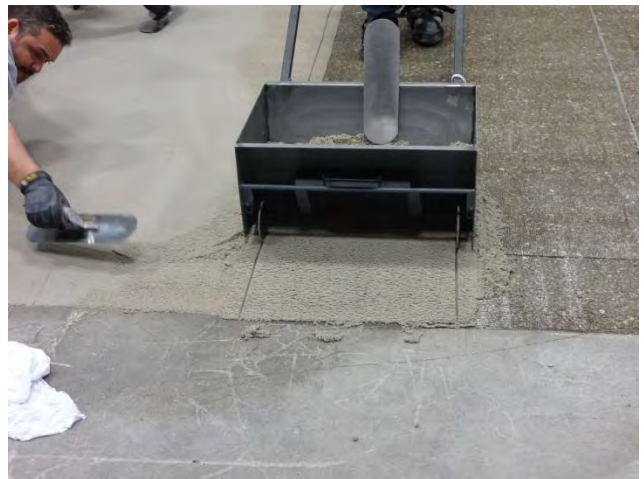
Troweling AH HDR behind the screed box
