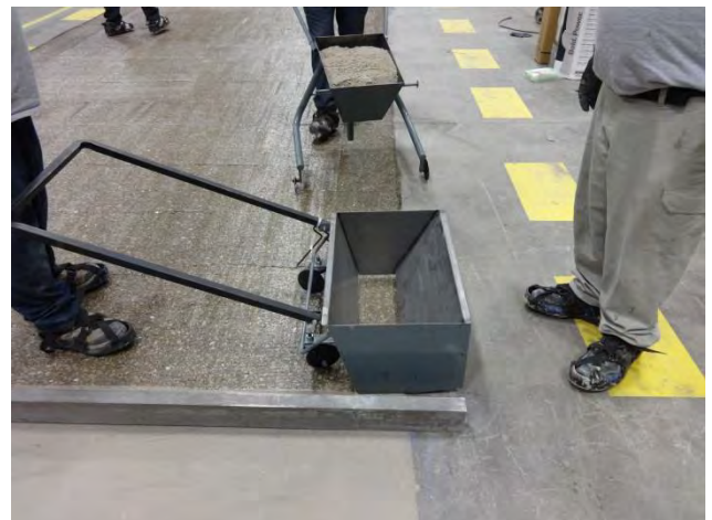
Preparing to place AH HDR into screed box
