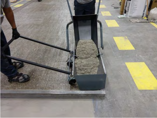
Dumping AH HDR mortar into screed box
